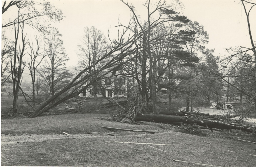
Route 20 and Warren Road
