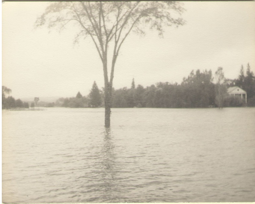
Looking toward Wales Road
