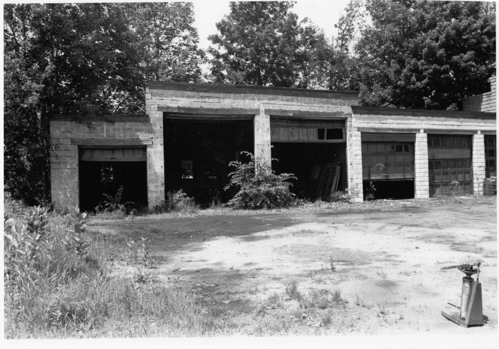
East side, bays at rear of building, July, 1976 (John Curtis, photographer)
