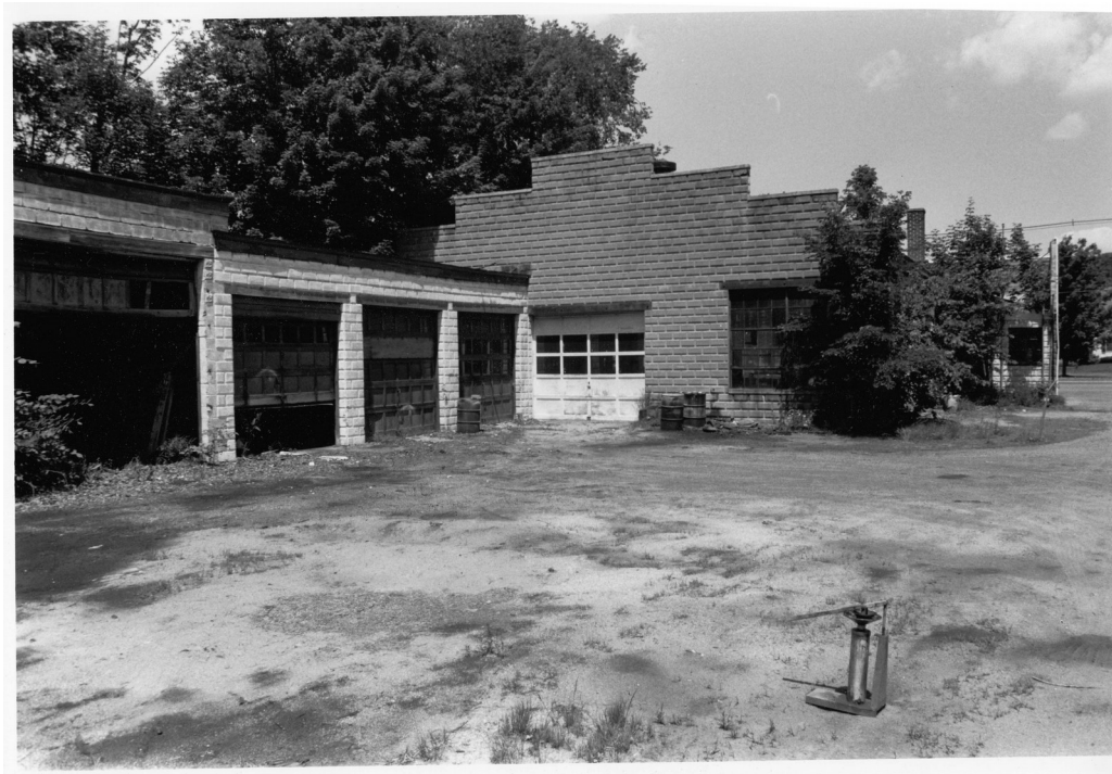
Rear of building, July, 1976 (John Curtis, photographer)
